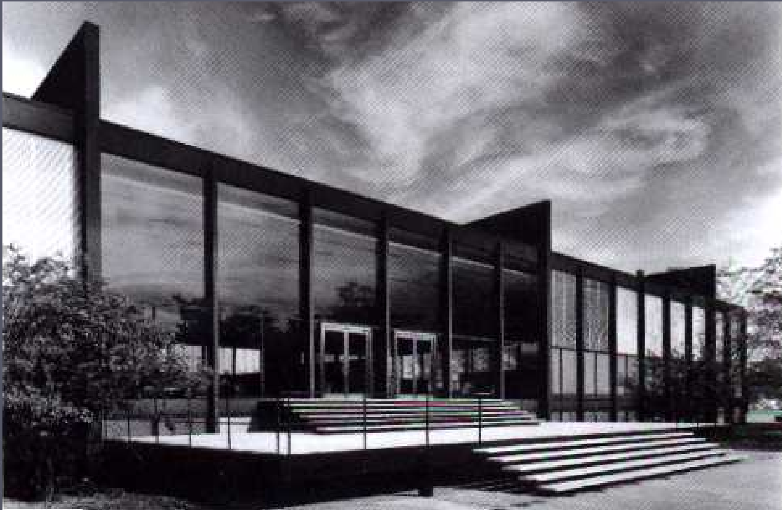
LUWING MIES VAN DER ROHE, Crown Hall, Illinois Institute of Technology, Chicago,
